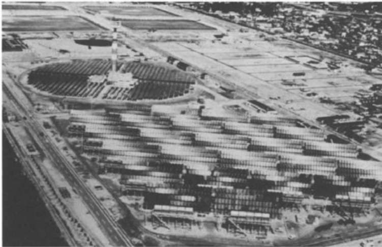
Fig. 1. A pilot 1 MW solar thermal power plant.
